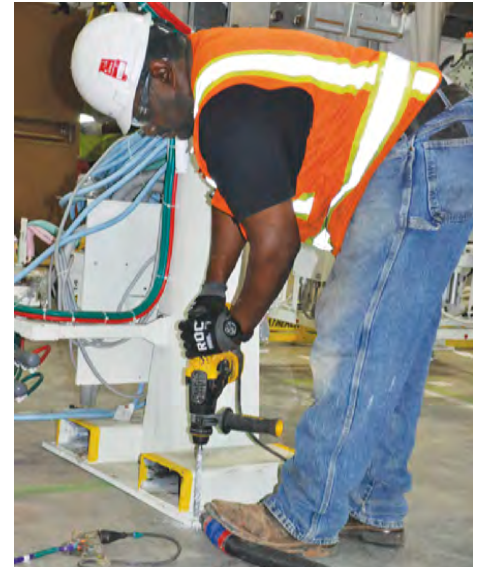
LEFT: Millwrights are installing all processing equipment, including conveyor systems and robots that will paint and weld body panels. RIGHT: Local 1192 member Milton Shelton anchors a robot base in the Toyota welding area of the plant.
